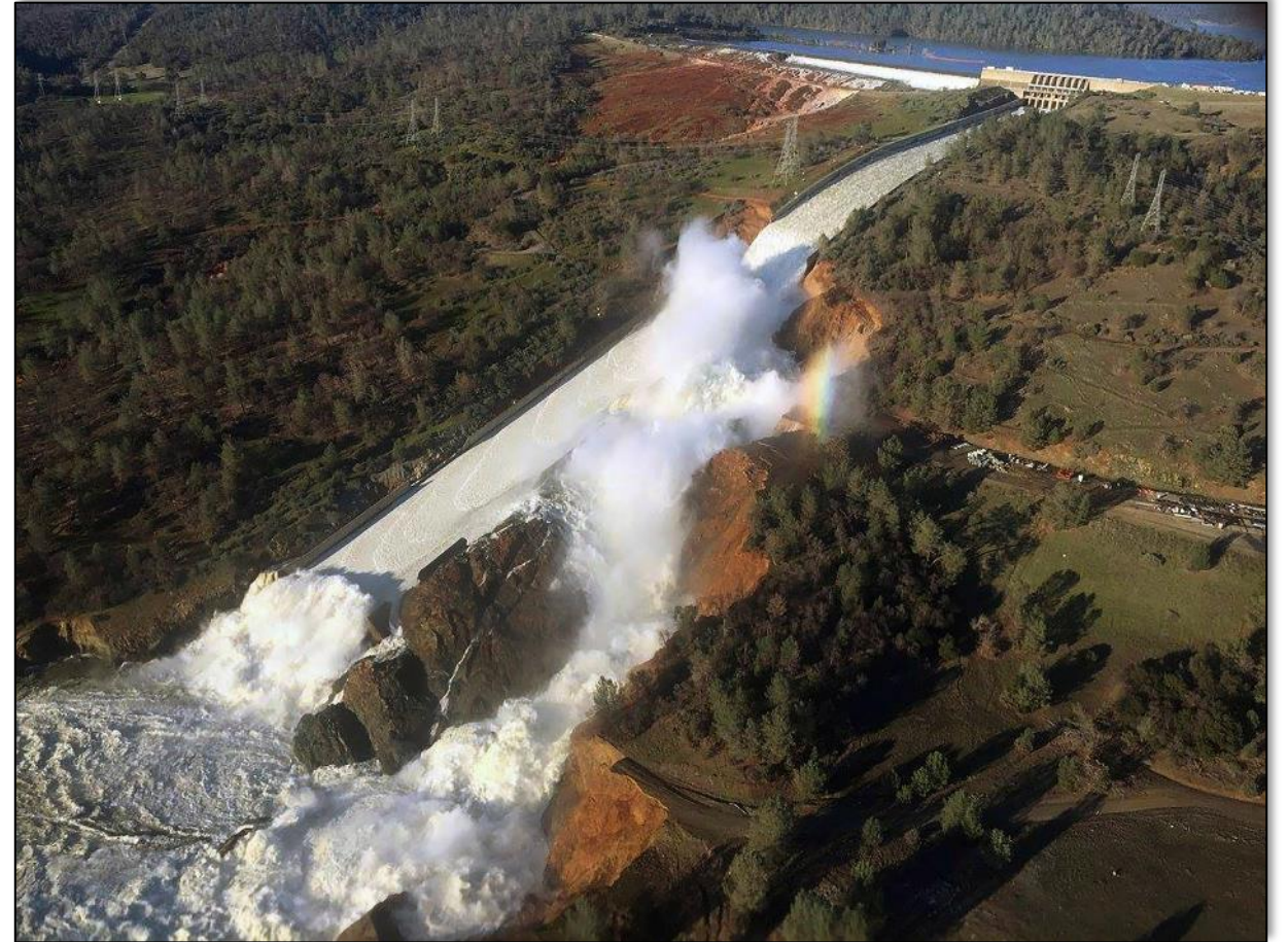
Oroville, CA Dam and Spillway Feb 2017 Photo credit: Public Domain
